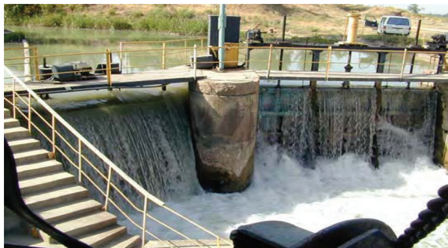
Figure 2.2. A small hydropower plant on the Alamedin River
