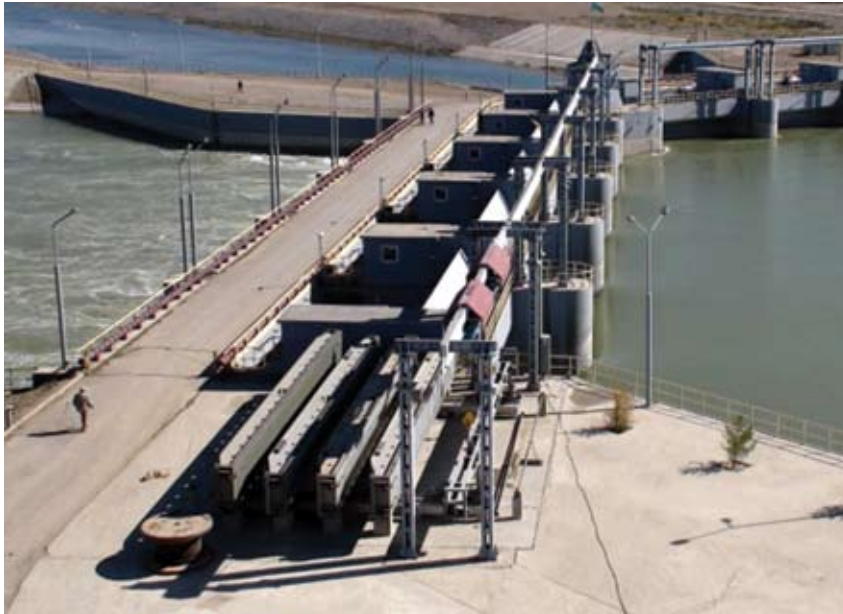
Figure 3.1 Headworks of the Koksaray Counter Regulator
